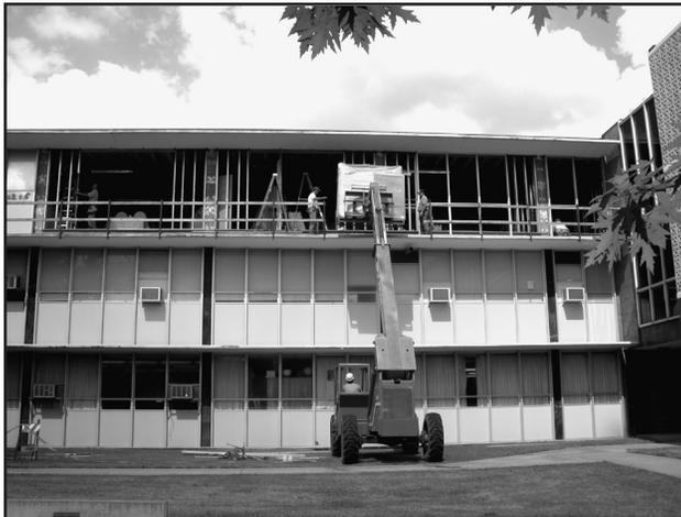
Workers prepare to install new energy-efficient windows and walls on the south side of the middle wing. Yes, it was completely open.
